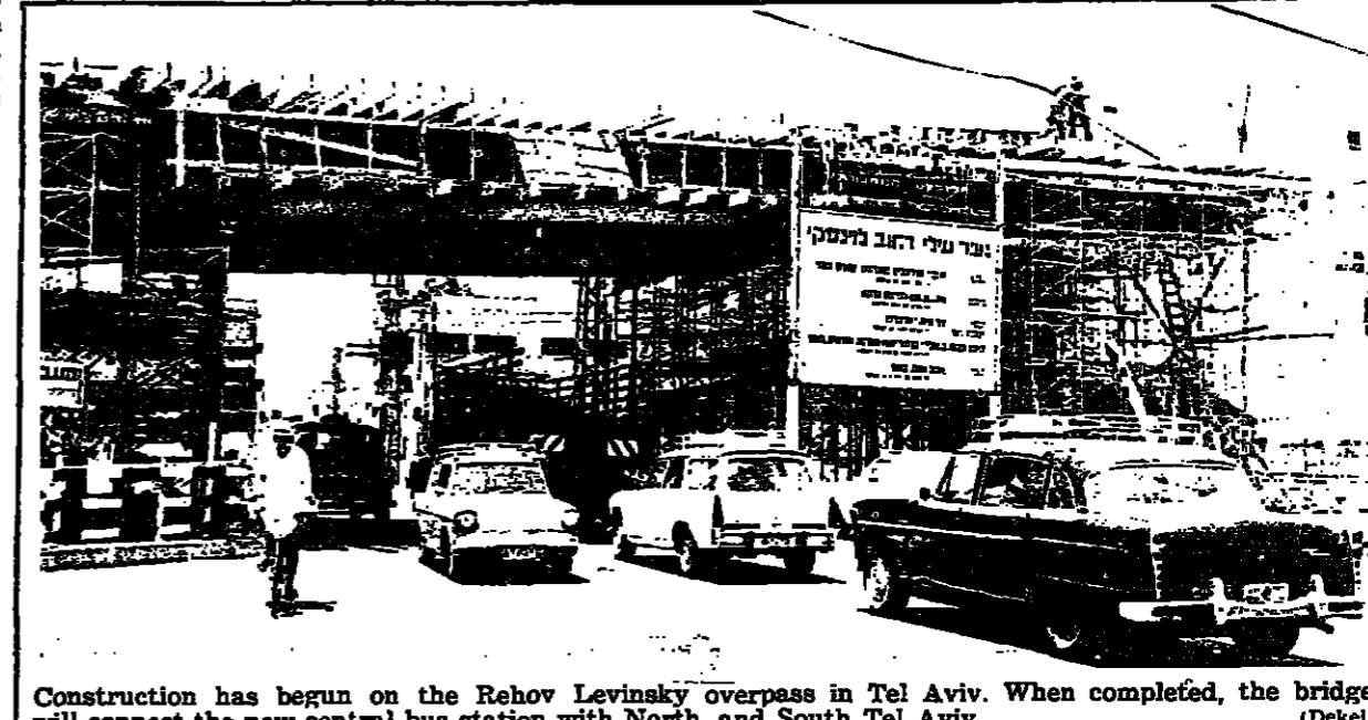
Construction has begun on the Rehov Levinsky overpass in Tel Aviv. When completed, the bridge will connect the new central bus station with North and South Tel Aviv. (Dekel)
